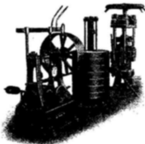
Fig. 10. — IMPIANTO IDRAULICO COMPLETO (POMPA 350 LITRI) PER LA FABBRICAZIONE DELLE PIASTRELLE COLORATE DA PAVIMENTO.
